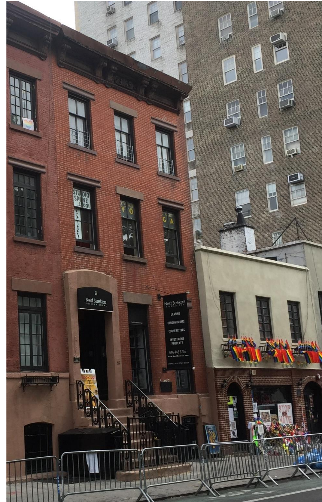
EXISTING CONDITIONS 55 CHRISTOPHER ST for which LPC Violation (16/1069) was issued for non-compliant plaques & banner. The need for commercial identification by commercial tenants and the placement of additional signage within the building behind the plane of the glass lends a haphazard and inconsistent appearance detracting from the historic character of the building.
